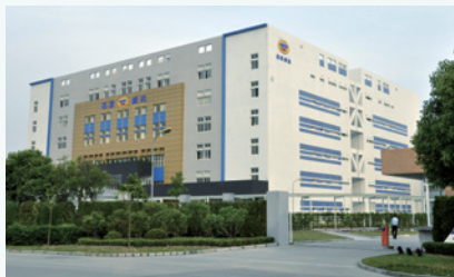
Armolink Site in Shanghai, China
